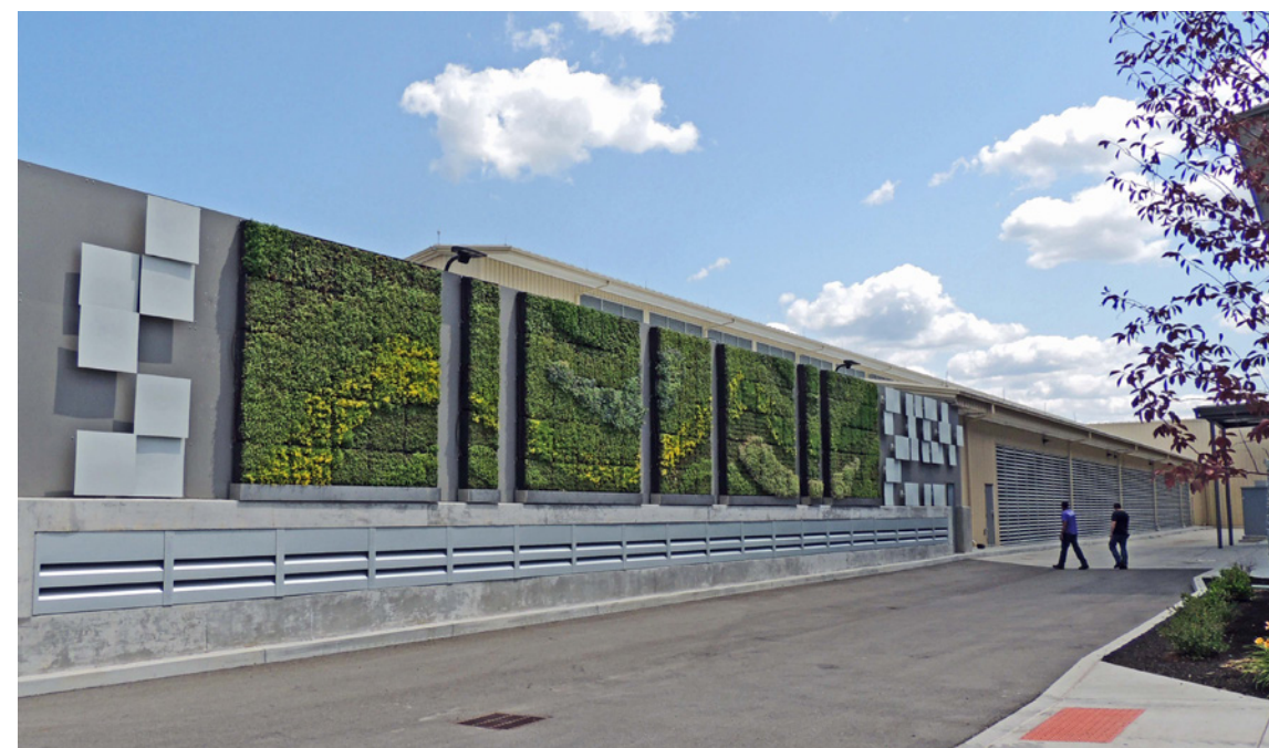
Yahoo's Compute Coop data center takes advantage of direct evaporative cooling.
