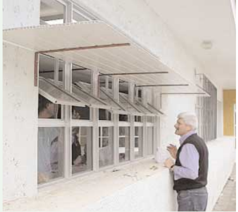
Above: Editor's pick for Best Action Photo: RMI's animated architect Huston Eubank explains the benefits of high-performance design to Governor Jaime Lerner of the state of Paraná, Brazil (note the fast-moving finger). Right: Lightshelves are easy to install, affordable by any society, and provide some of the greatest benefits to students and faculty. The exterior lightshelf shades the glass below it, while both it and its interior extension bounce daylight up onto the ceiling.
