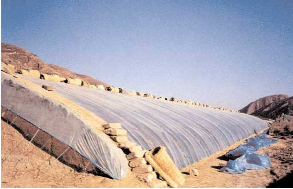
Passive solar greenhouses such as this have extended the growing season in Western China, expanded the crop mix, and improved the income of remote villages.
