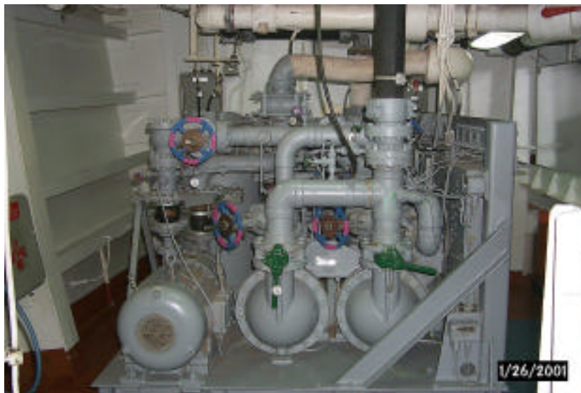
Equipment cooling heat exchanger. Ron Perkins photo.
