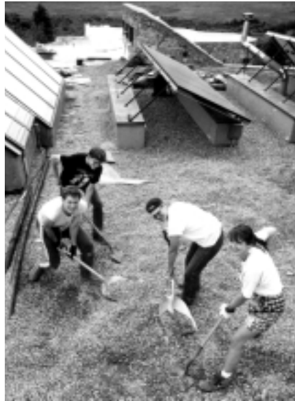
Digging in: André, Franz, Ruth, and Kate clear gravel from the old roof.
