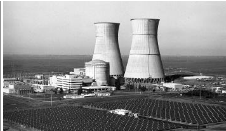
George Turner, SMUD Changing times: The Sacramento Municipal Utility District has erected a grid-connected array of PV panels on the grounds of its now-abandoned Rancho Seco nuclear power plant.
