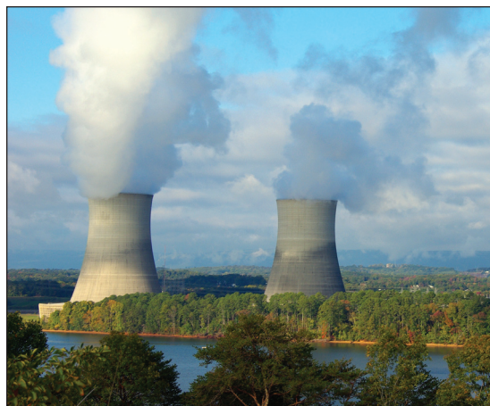
The Sequoyah nuclear generating station, near Chattanooga
