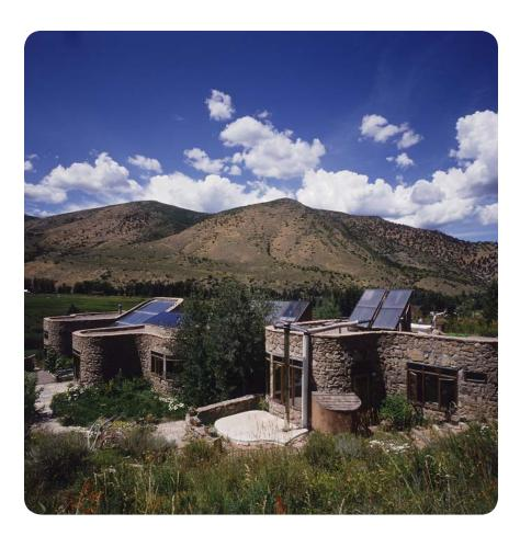
and partly for backup heating. The passive solar design also incorporates daylighting and natural ventilation while preserving viewlines and minimizing noise.
