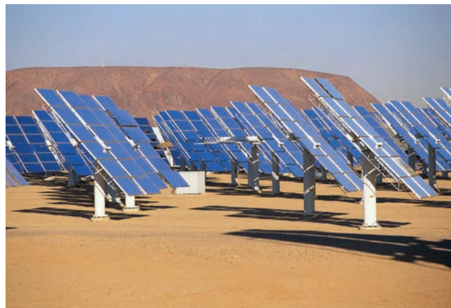
ERT continues its work on Next Generation Utilities.
