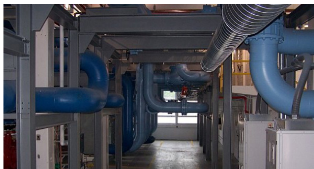
Effluent heat exchange facility at the main base Image courtesy of: Trane U.S., Inc.
